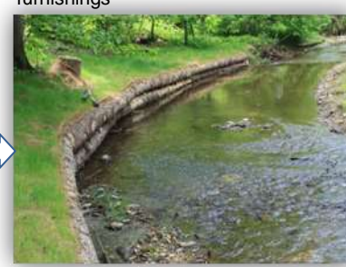
After: stream bank restoration
