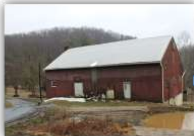
Before: stormwater issues
